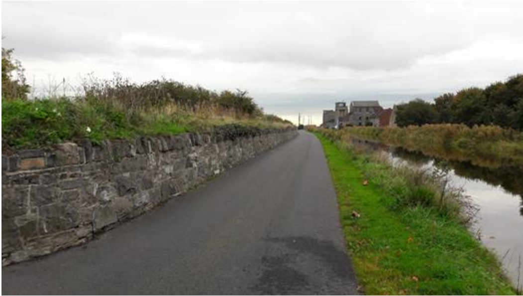
Fig. 4: Existing view of Section 3: Looking eastward from Coke Oven Cottages.
