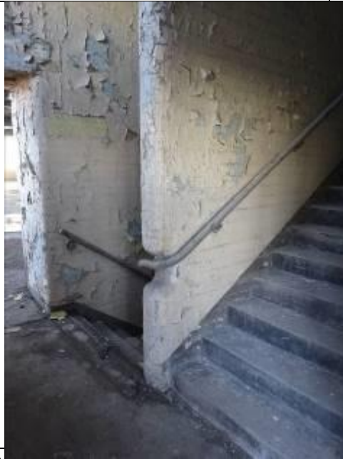
Fig 11: Concrete staircase to east with handrail recess
