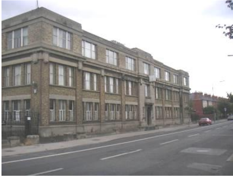
Fig 3: South elevation from southwest
