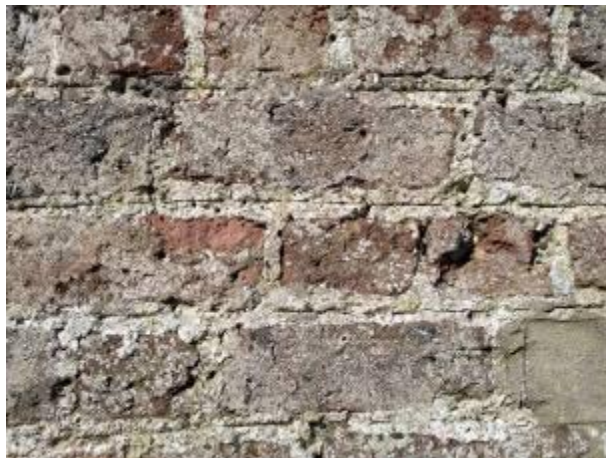
Note surviving penny struck lime mortar joint.
