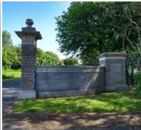
View of southwest side of Neoclassical Northern Gateway, with curving ashlar wall with tall elegant gate-pier and curving ashlar wall terminated by a squat, wide pier. Gate piers display vermiculated rustication.
