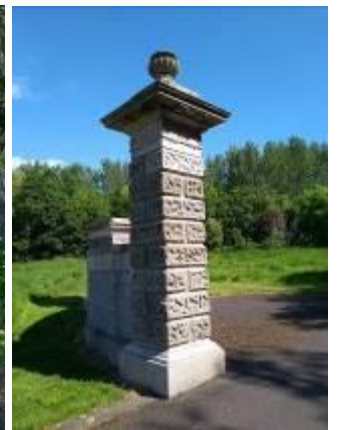
View of southwest side of Neoclassical Northern Gateway, with curving ashlar wall with tall elegant gate-pier and curving ashlar wall terminated by a squat, wide pier. Gate piers display vermiculated rustication.
