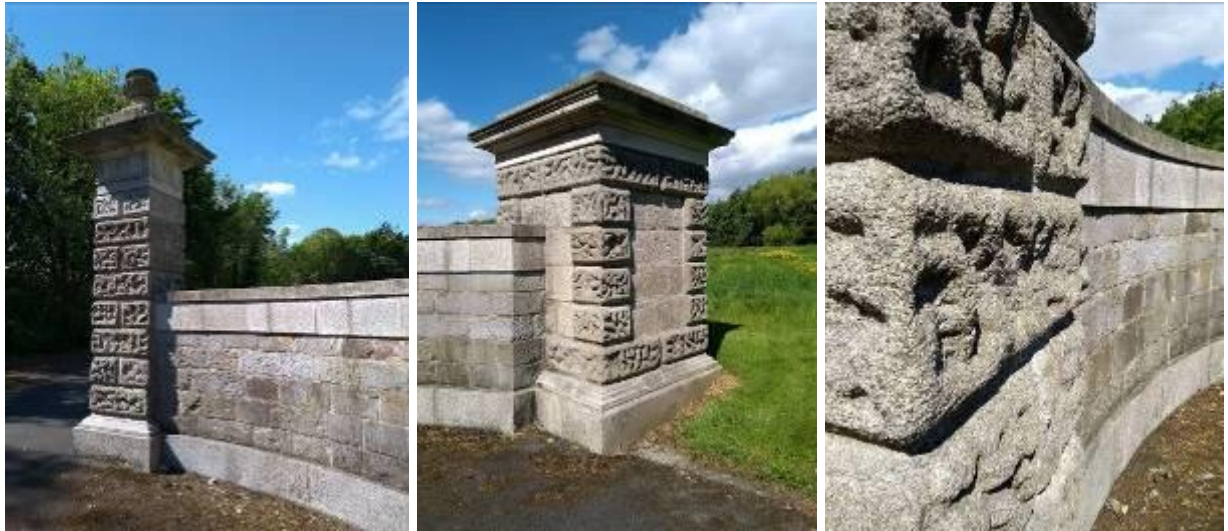
Detail of tall elegant gate piers to left topped with urns on a swag-enriched plinth, which sit on ornamental cappings with Doric enrichments and bucrania identical to those of the outer piers of the Griffin Gateway. The different materials used - limestone and granite clearly visible.
