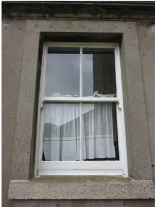
Fig.9: Two-over-two sliding sash window having ogee horns to link corridor to north and west of chapel representing surviving historic timber sashes.
