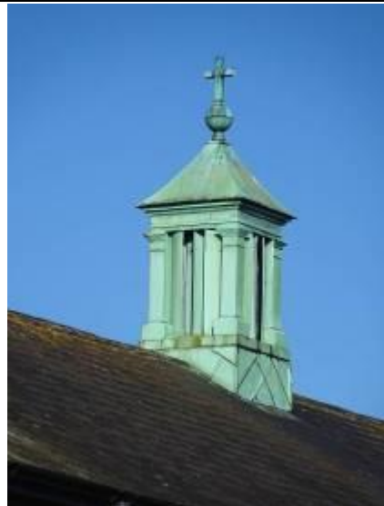
Fig.6: Copper-clad lantern surmounted by cross finial to centre ridge of chapel.
