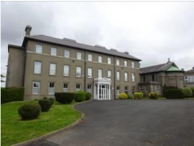
Fig.3: Principal elevation of convent with chapel to right of image.
