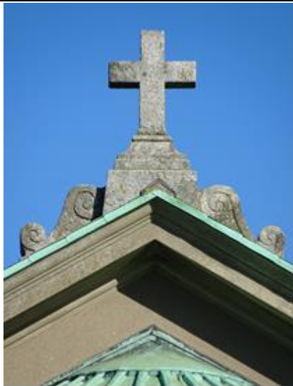
Fig.5: Granite cross finial to gable apex of chapel.
