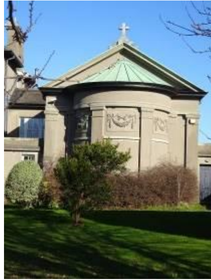
Fig.4: Semi-circular apse to chapel with copper-clad roof and giant order of Doric pilasters.
