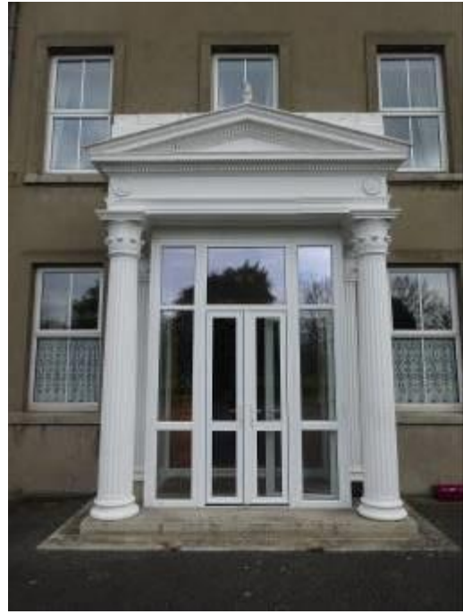
Fig.10: Painted stone portico (Portland limestone) with lotus leaf capitals, now with glazed porch inserted.
