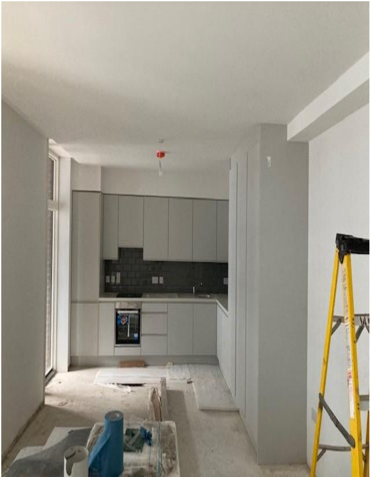
Fitout works ongoing in the apartments.
