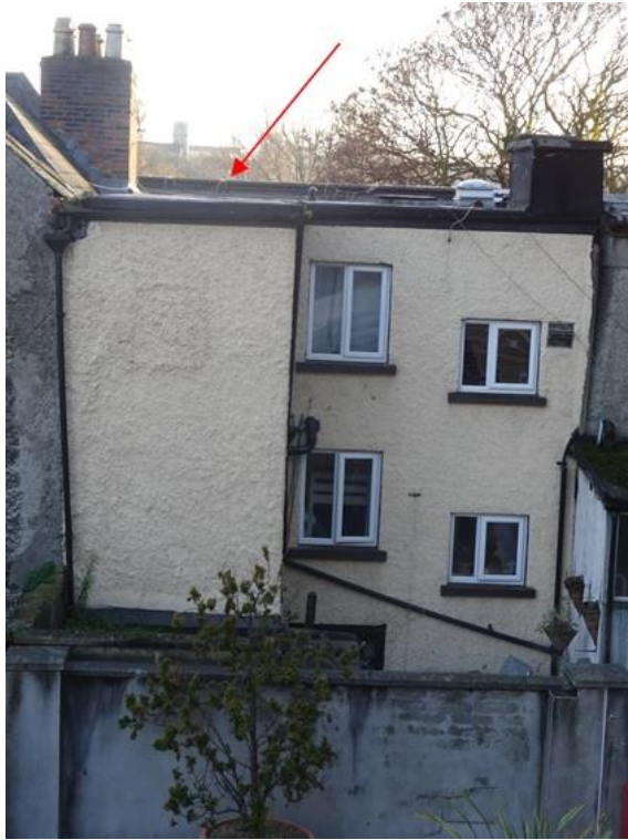
Fig.6: Rear aspect of No.7 showing closet return (arrowed) indicative of an early date. Note the externally mounted water tank to right of roof.
