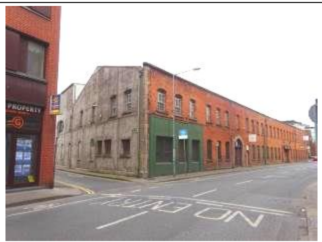
Fig 3: View from northeast
