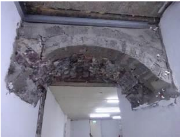
Fig 18: Arch to opening in basement containing historic fabric
