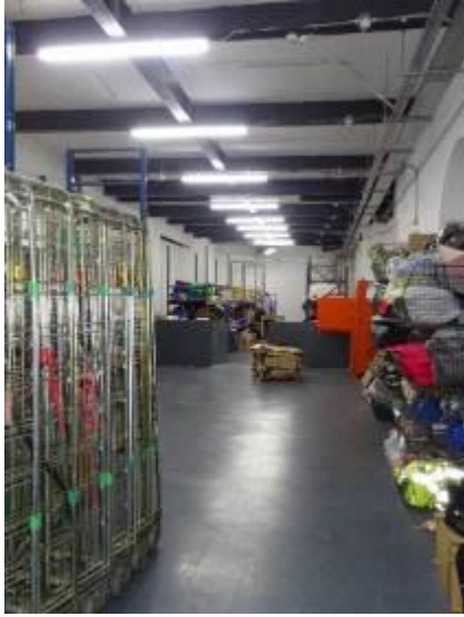
Fig 14: Ground floor, east end of structure looking south
