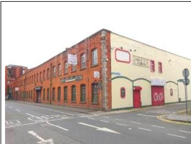
Fig 2: View from northwest
