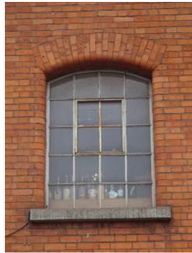
Fig 9: Metal window, north elevation
