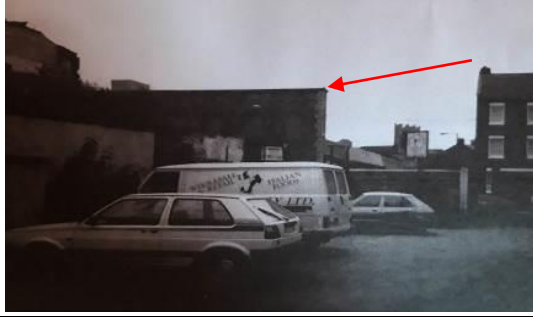
Fig 24: Image dated c.1990 with two-storey façade to northwest corner of 139-149 North King Street arrowed red; note single-storey structure behind
