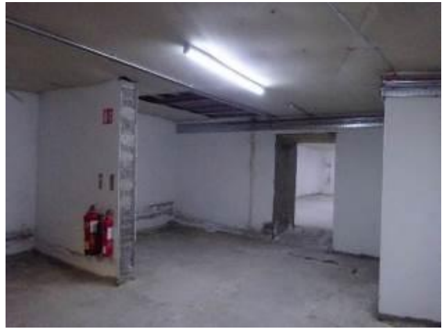
Fig 17: View of section of basement looking south
