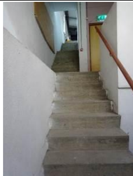
Fig 13: Concrete staircase from ground to first floors
