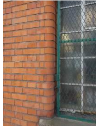
Fig 11: Detail of brickwork to openings, north elevation
