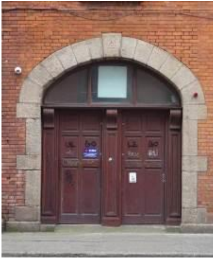
Fig 10: Former goods entrance, north elevation
