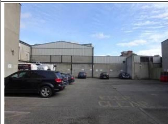
Fig 6: West elevation of N-S running section of building along Bow Street
