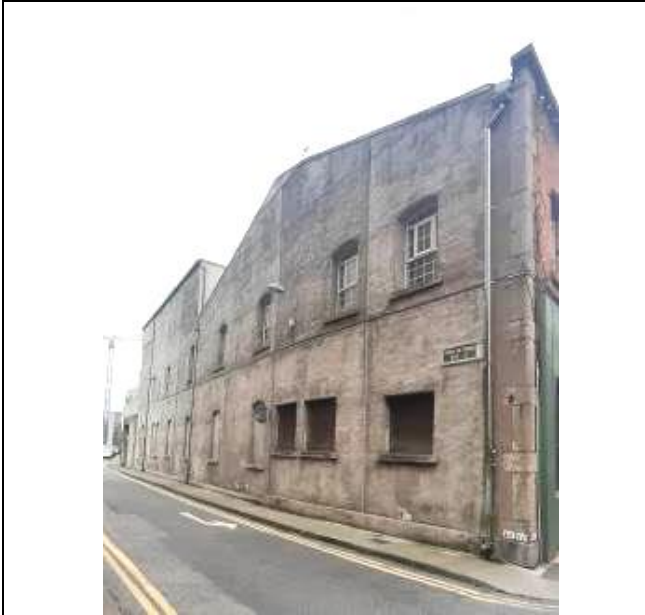
Fig 4: East elevation from northeast
