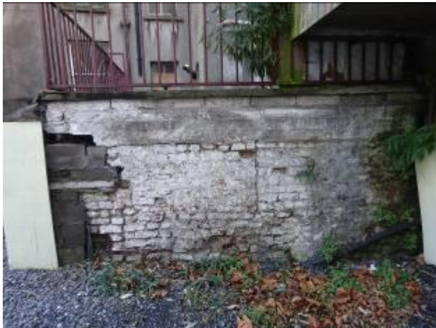
Fig.8: Surviving section of brick wall forming party boundary with No.4 and 5 Parkgate Street.
