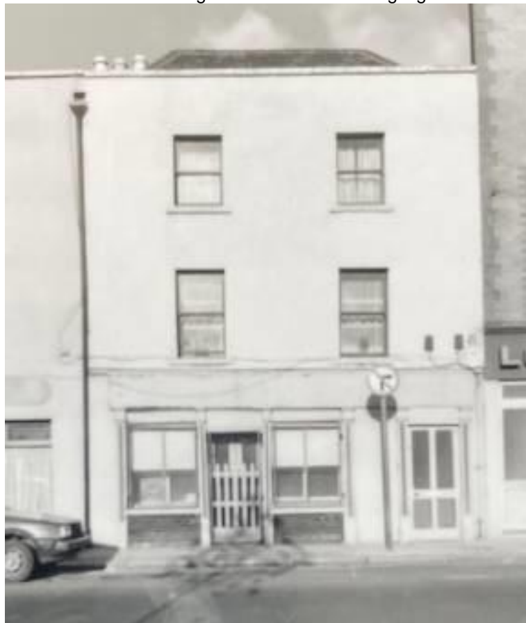
Fig.14: No.6 Parkgate Street c.1970 showing the modest shopfront (Image Courtesy of the IAA).
