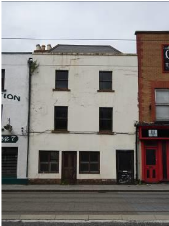
Fig.3: Principal/south elevation. Note the steeply pitched hipped roof, substantial chimney stack & disproportionate ratio of solid to void to the elevation indicating an early construction date.
