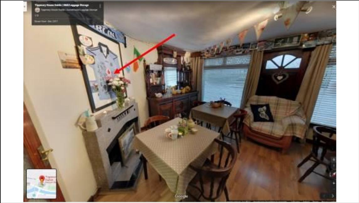
Fig.14: Image of ground floor front room. Note the low floor to ceiling heights, substantial corner chimney breast (arrowed red) and the former shop display windows and separate shop door access.
