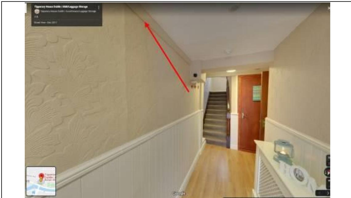
Fig.12: Image showing ground floor entrance hall. Note the moulded cornice to the west wall (arrowed).
