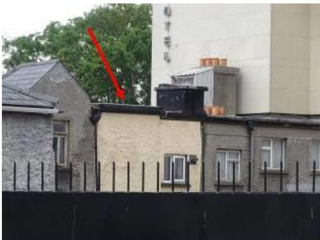
Fig.6: Rear aspect of No.7 showing closet return (arrowed) indicative of an early date.
