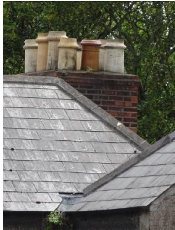
Fig.7: Detail of substantial chimney stack shared with No.7 Parkgate Street.
