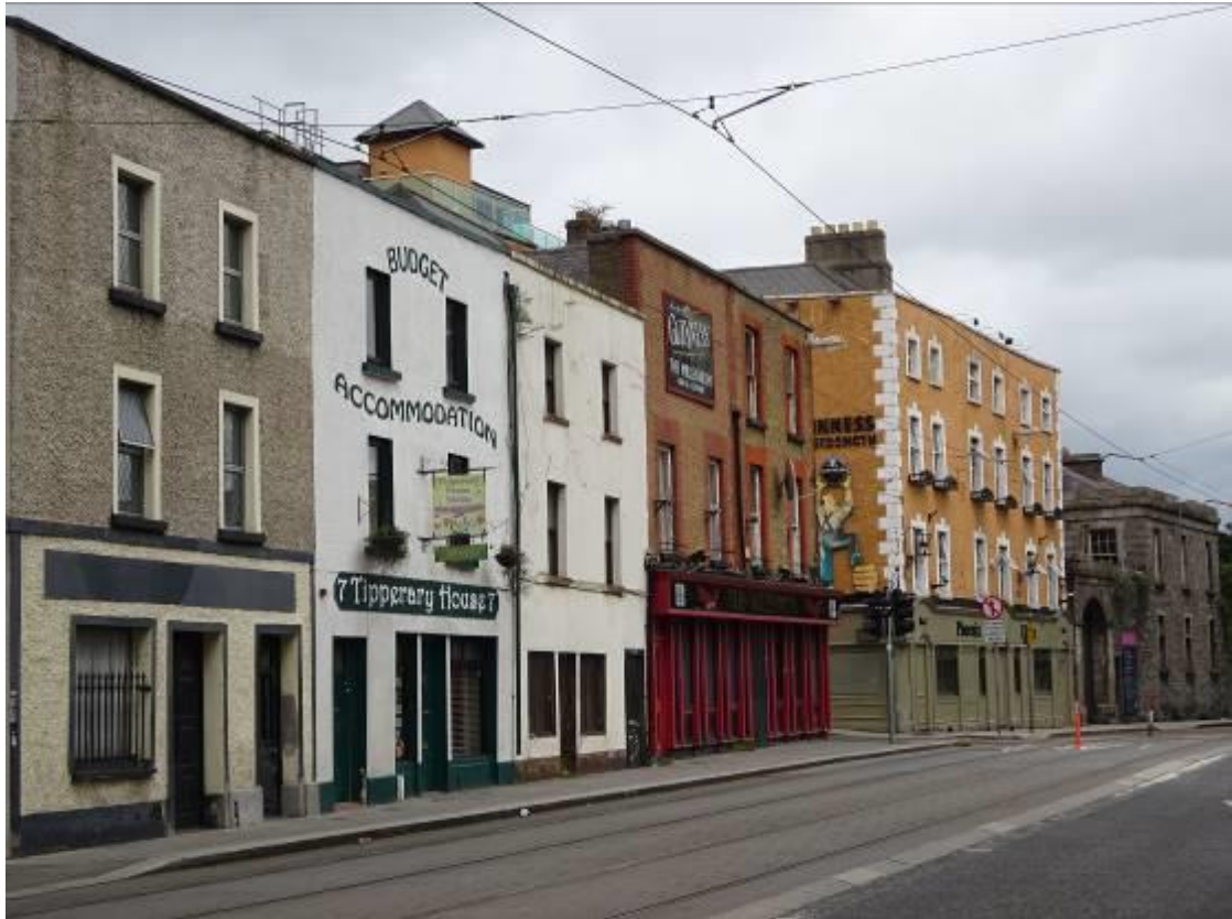
Fig.5: Context view of No.6 Parkgate Street taken from the west showing part of the National Museum of Ireland, Collins Barracks to the extreme right of image.
