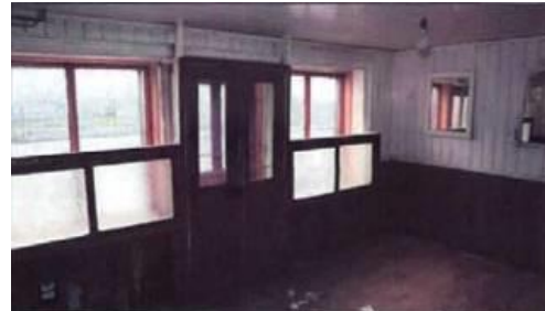
Fig.22: Aspect of ground floor shop. Note the timber sheeted walls, double-leaf doors and horizontal sliding glazed screens to display windows.
