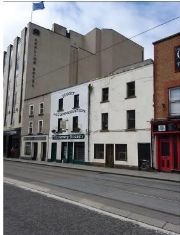
Fig4: Context view of No.6 (right), No.7 (centre) and No.8 (left) Parkage Street taken from the east showing the properties dominated by the Aisling Hotel.
