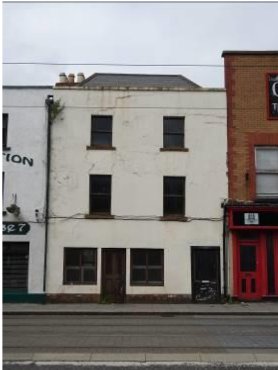
Fig.3: Principal/south elevation. Note the steeply pitched hipped roof, substantial chimney stack & disproportionate ratio of solid to void indicating an early construction date.
