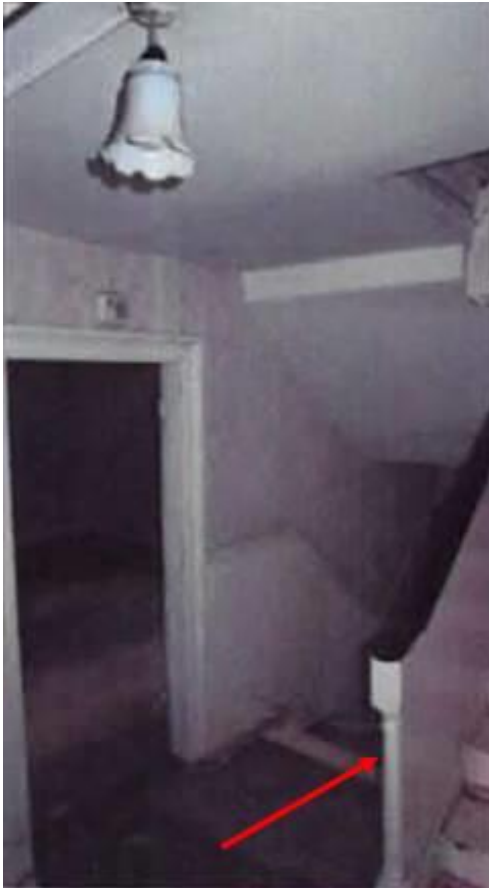
Fig.13: Image showing first floor landing. Note the Doric newel post and ramped banister rail typical of the early-to-mid 18th century (arrowed). Also note the moulded timber door architrave.
