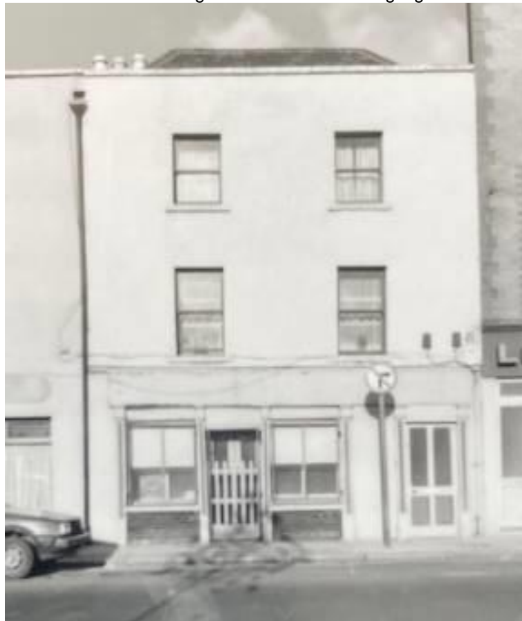
Fig.12: No.6 Parkgate Street c.1970 showing the modest shopfront (Image Courtesy of the IAA).
