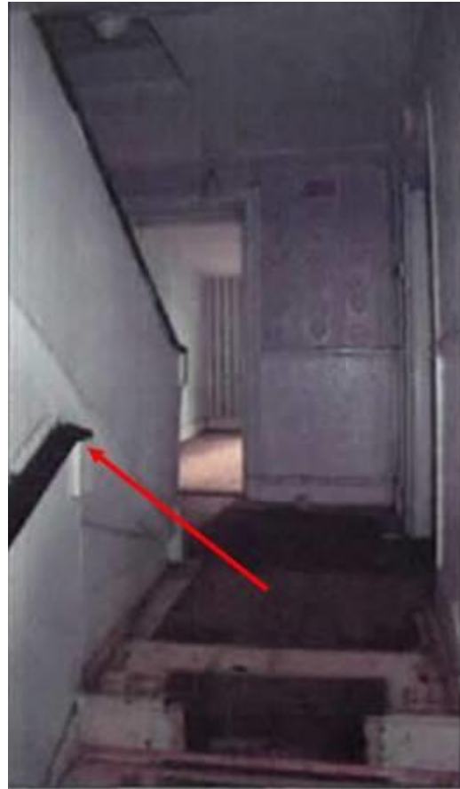
Fig.14: Detail of first floor landing showing intersecting handrail typical of the early-to-mid 18th century (arrowed).
