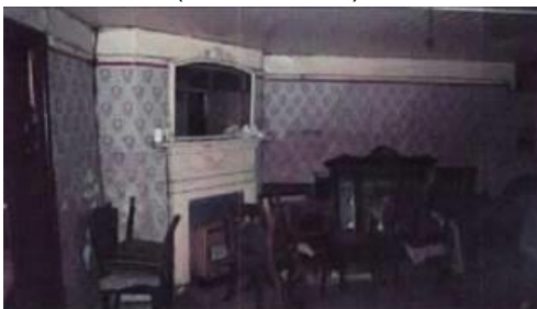
Fig.17: Aspect of ground floor rear room. Note the substantial corner chimney breast
