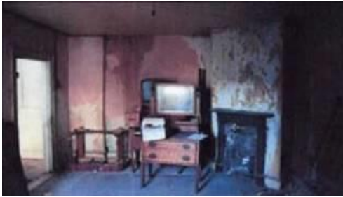
Fig.21: Aspect of second floor rear room. Note the corner chimney breast with cast-iron fireplace.
