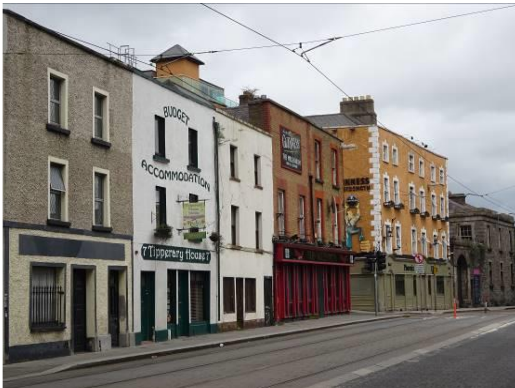
Fig.5: Context view of No.8 Parkgate Street taken from the west showing part of the National Museum of Ireland, Collins Barracks to the extreme right of image.
