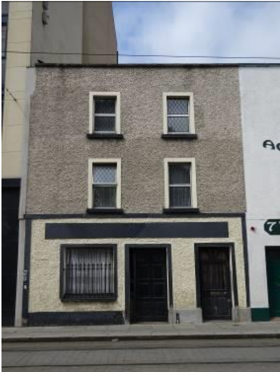
Fig.3: Principal/south elevation. Note the disproportionate ratio of solid to void indicating an early construction date.
