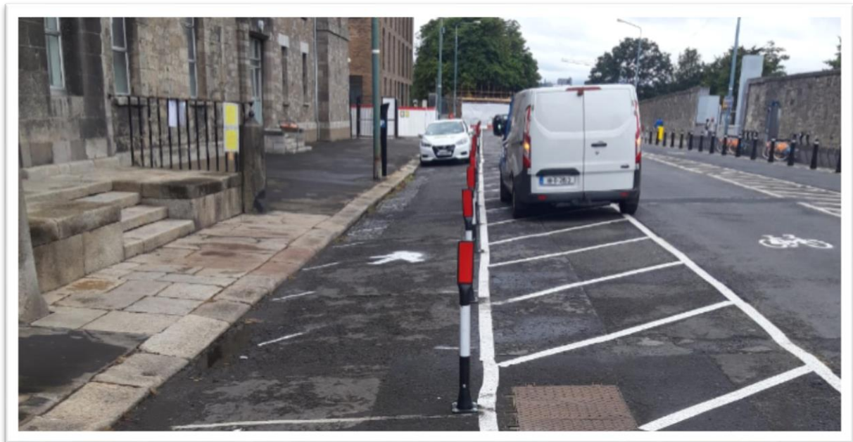
Figure 3. Additional Pedestrian Space (under construction)
