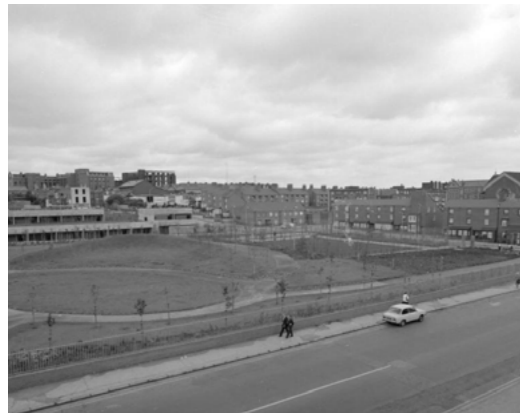
Above: Diamond Park under construction, Lord Mayor Bertie Ahern opens Diamond Park in 1986, looking north east over Sean MacDermott Street towards Gloucester Place (Dublin City Library Digital Collections).
