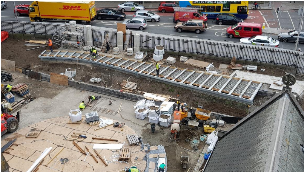
Image from roof of Christchurch Cathedral of works in progress
