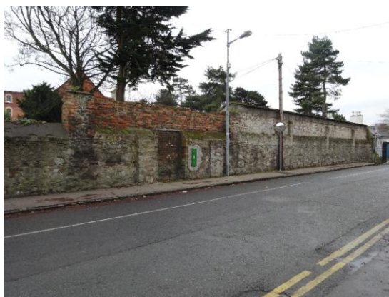
Structure 11: Rubble stone and brick boundary wall to Bloomfield Avenue.
