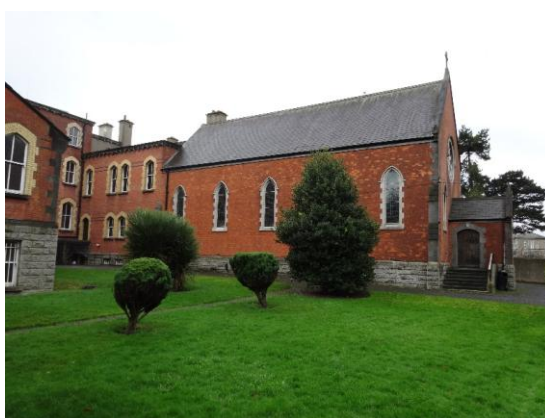
Structures 3 and 4 East-facing elevation of chapel and block to south
