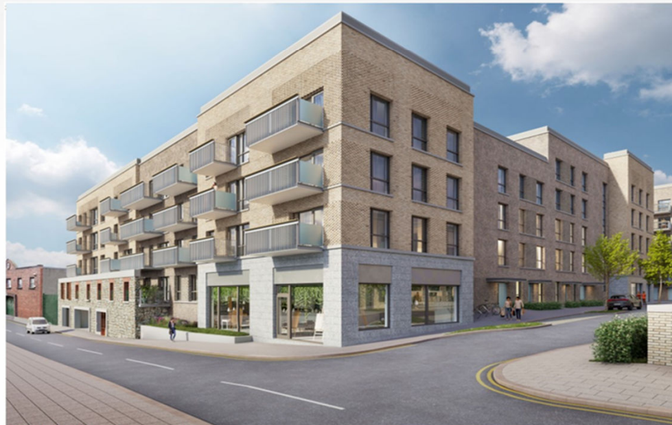
03 - View Looking South-West from Grangegoman Lower
