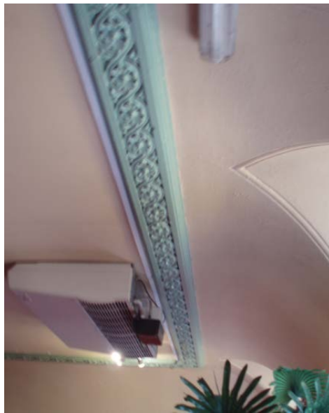
First floor plaster detail
