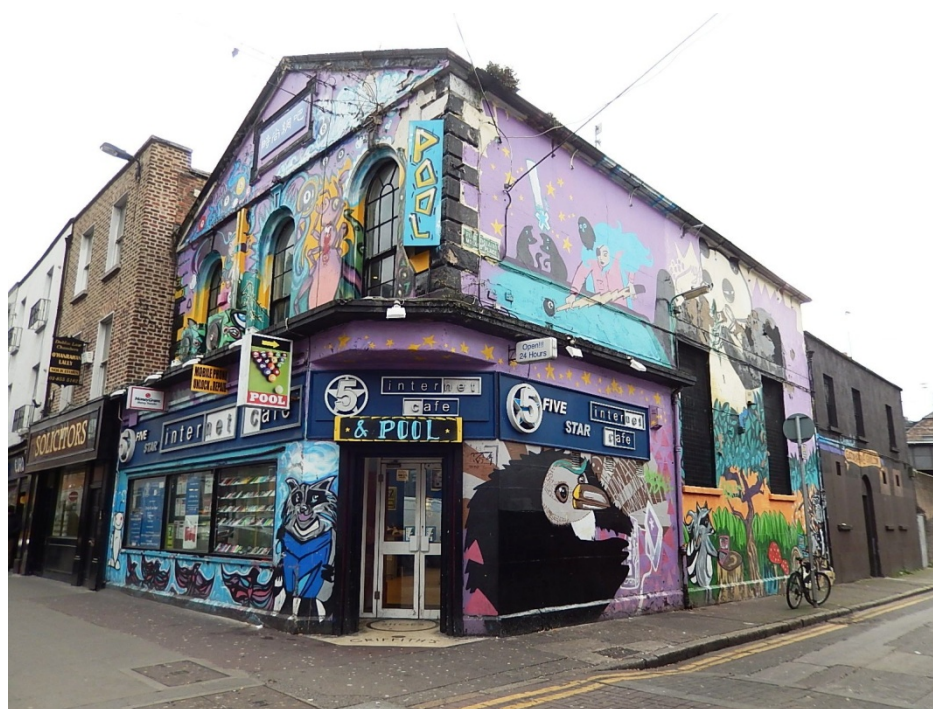
View of former Welsh Methodist Chapel (aka Old Welsh Chapel) on Talbot Street
