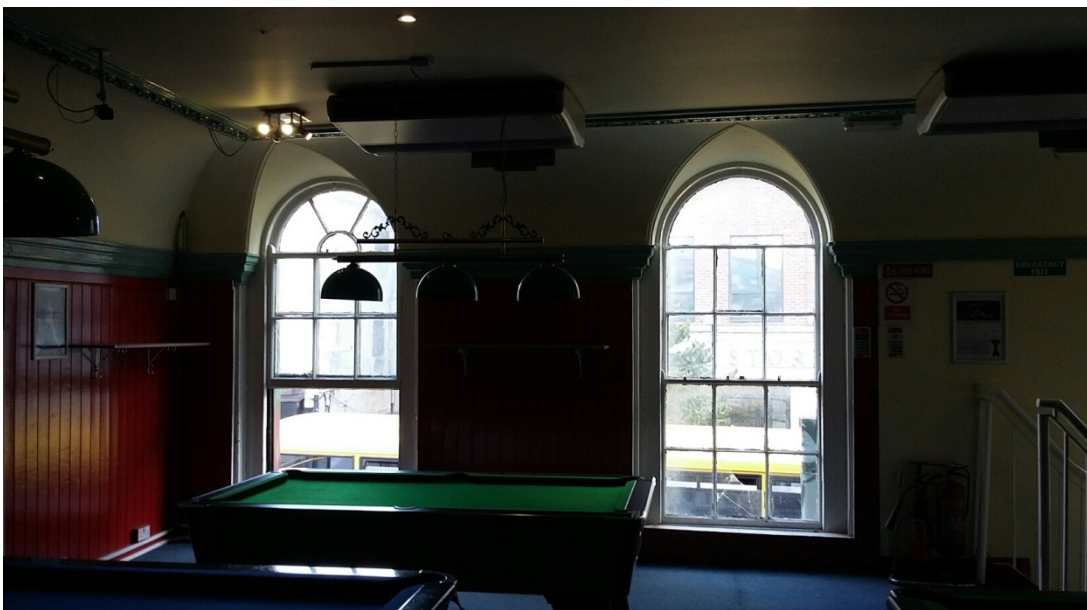
First floor interior – note: arched window openings and rounded sliding sash windows
