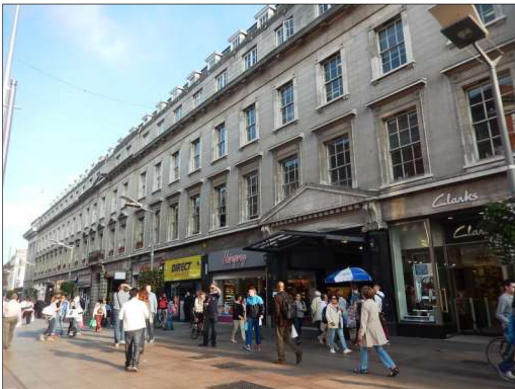
View of N side of GPO and 26-30 Henry Street
