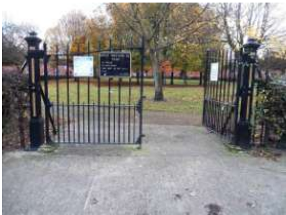
Historic entrance gate to N side of green space
