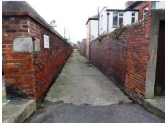
View of rear lane
