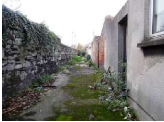
View of rear lane with calp limestone wall
