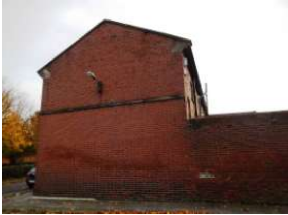
Gable detail of house on west side
