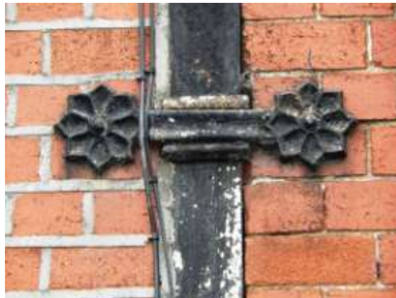
View of recessed cast-iron downpipe detail
