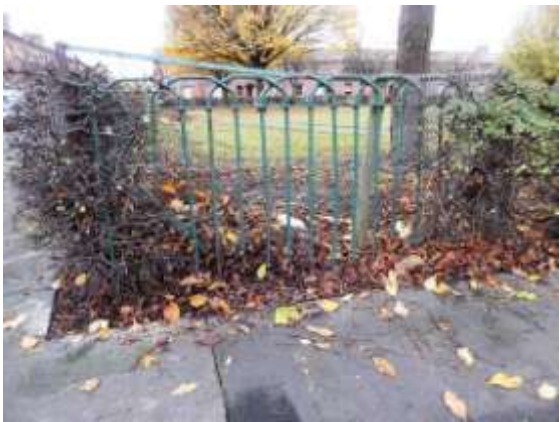
Section of earlier railings to SE corner
