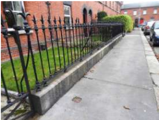
View of railings and gardens to front
