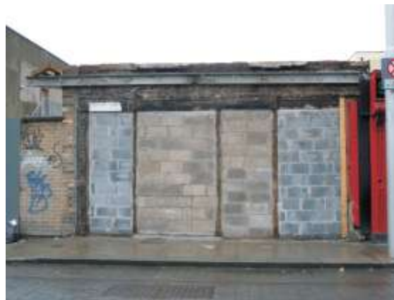
Figure 1: No. 6 Post demolition Photo: BAR Photographic Survey: 26/03/12
